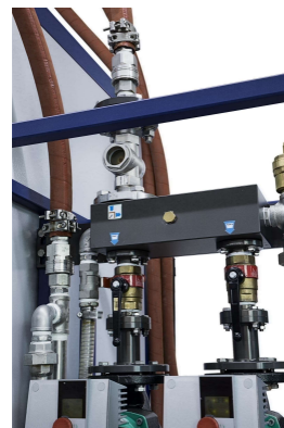
Separate Cooling Rack Configuration
